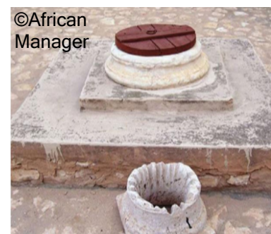
Photo 3: Majels, rainwater storage tanks in Tunisia
